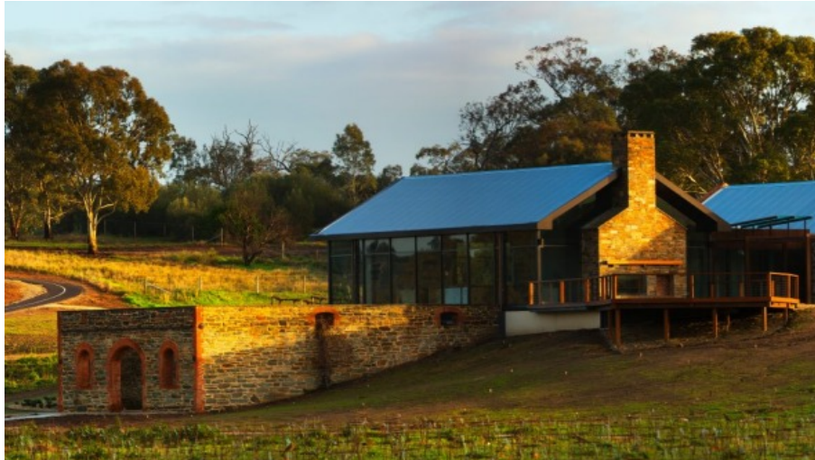
The home of St Hugo was built using the ironstone walls of a 1854 gravity-fed winery owned by the Gramp family. Dragan Radocaj
