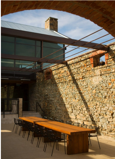
The ironstone walls of the new courtyard took six months to repaint. Dragan Radocaj
